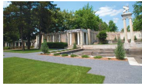
Untermeyer Park in Yonkers, NY— Stabilized Pathways
