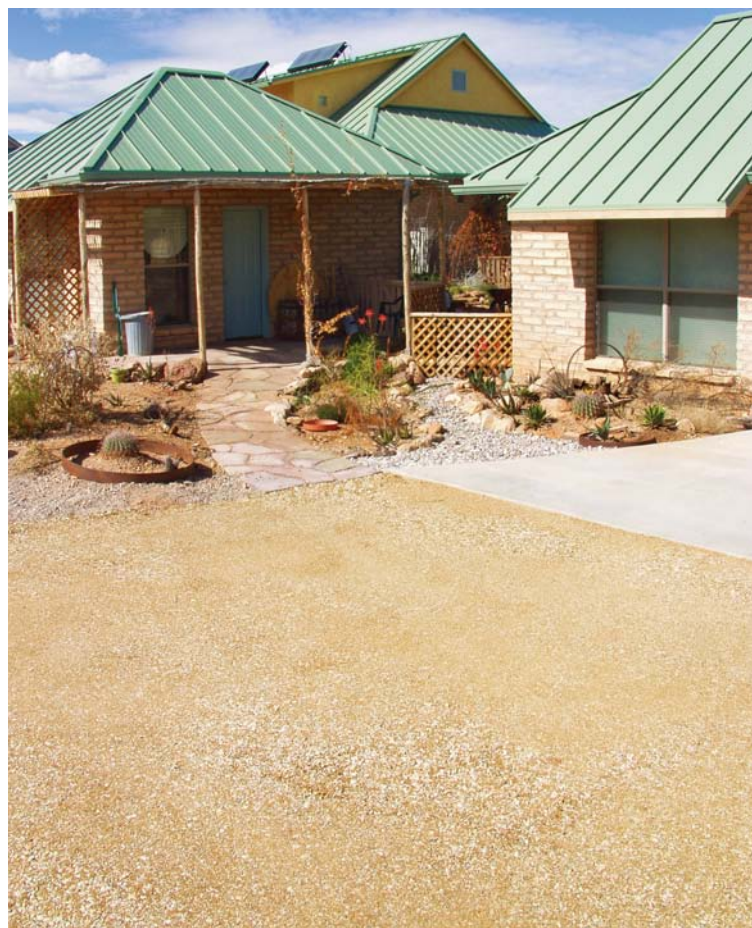
Milagro Co-Housing Project in Tucson, AZ—StaLok® Pathway Mix, Gold
